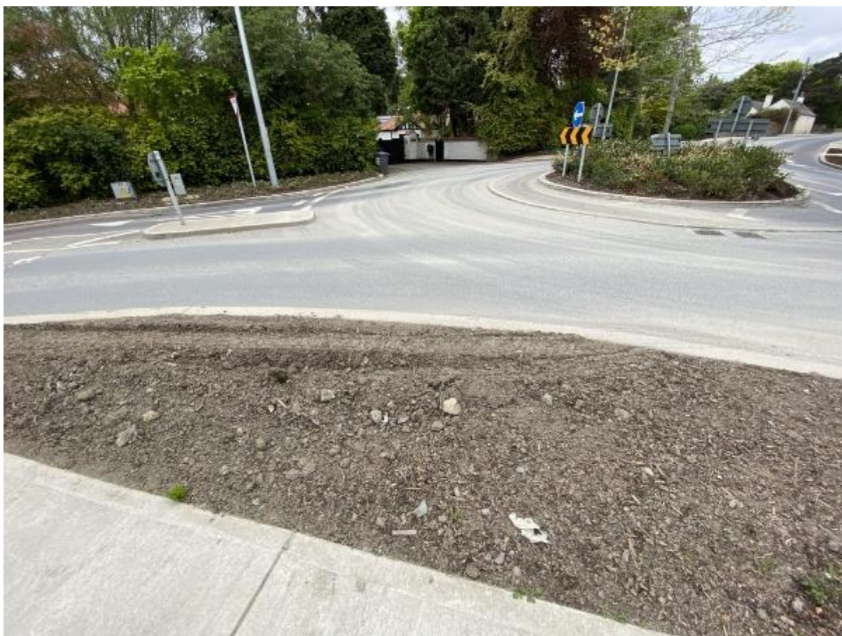
Figure 26 Photo 6 - New roundabout with evidence of vehicles mounting kerb
