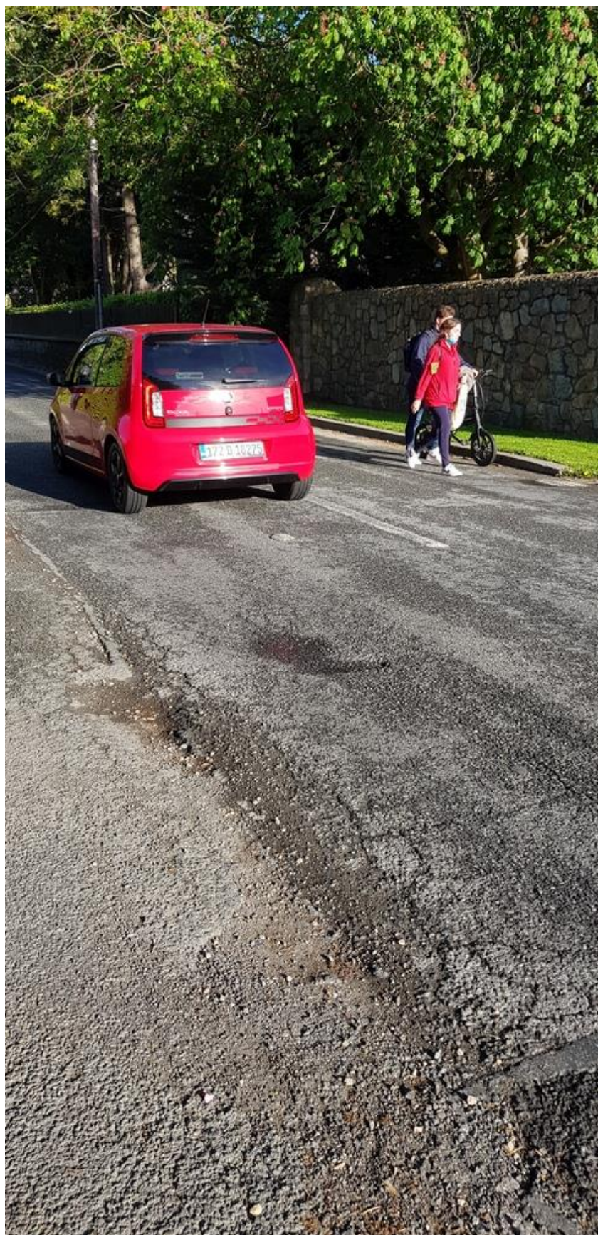
Figure 15 Pavement failure - Brennanstown Road
