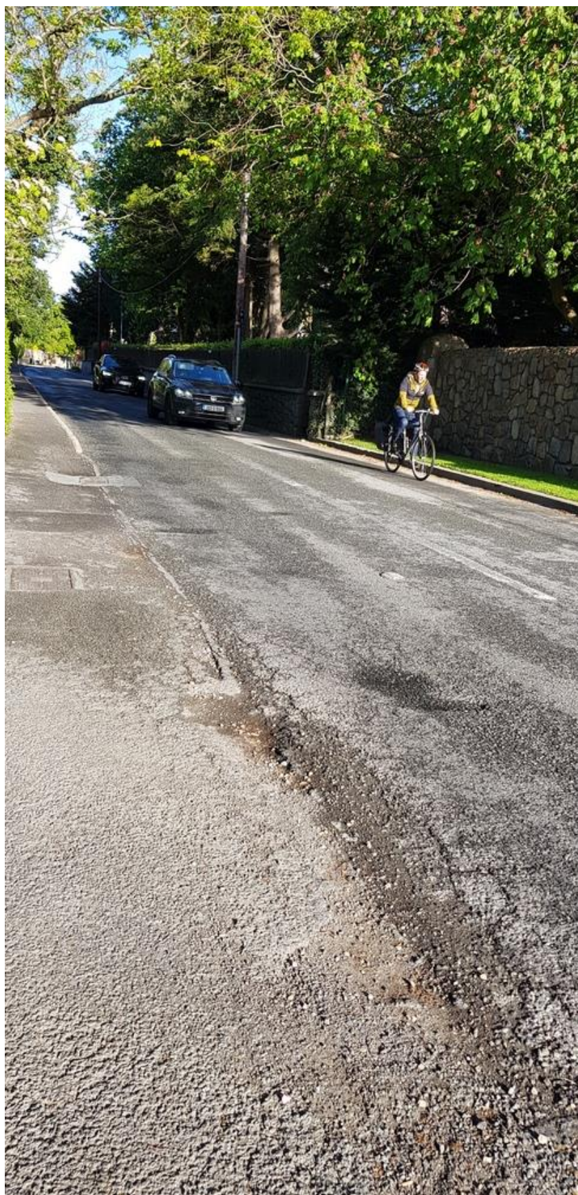
Figure 33 Photo 13 - Pavement failure - Brennanstown Road
