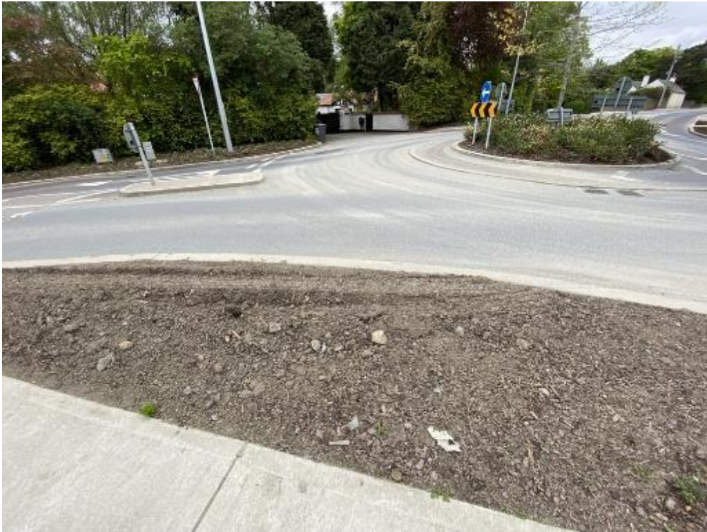
Figure 14 Kerb oversailing
